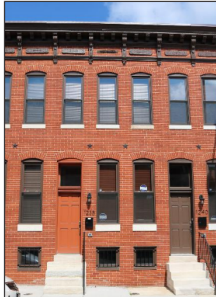
Figure 5: RECOMMENDED - Repointed brick that replicates the color, texture, composition, and tooling of the historic mortar.
