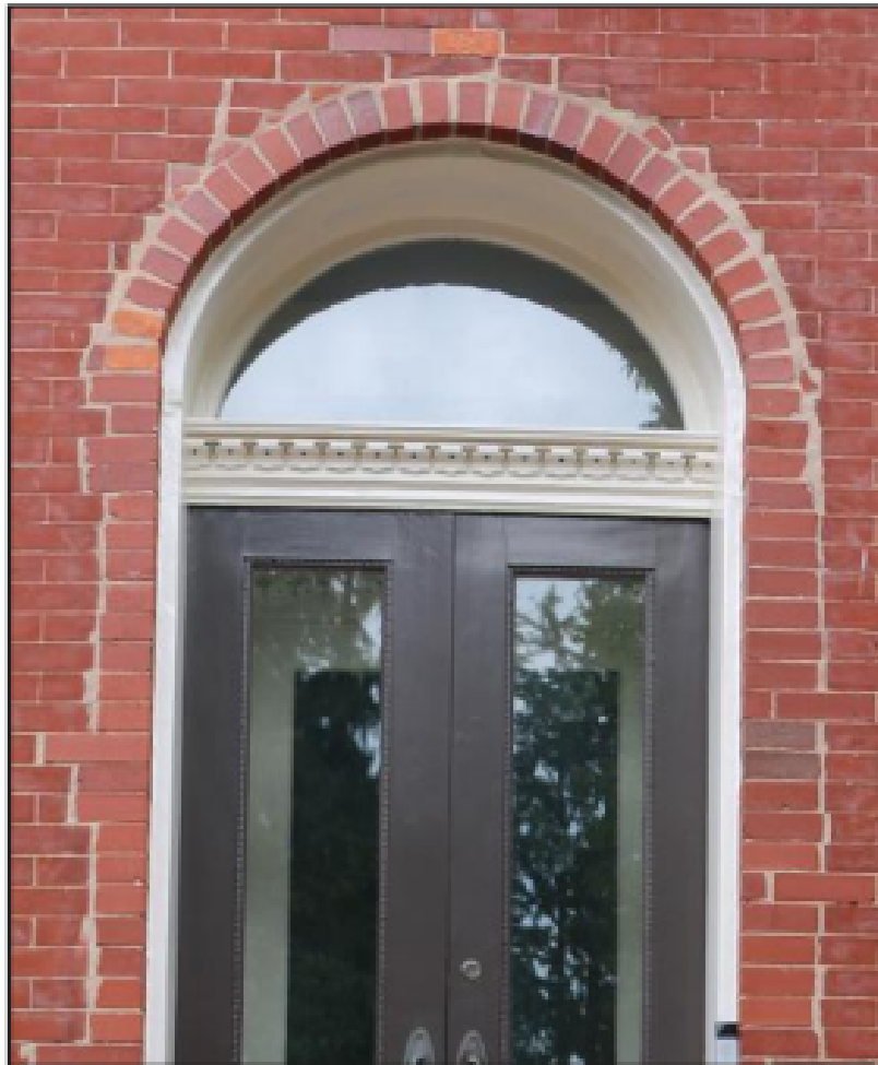
Figure 4: NOT RECOMMENDED - Inappropriate repointing following the removal of historic door surround.
